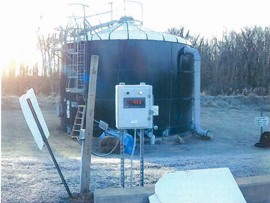
Date: 12/12/2011 Time: 7:47 a.m. Direction: southeast Photo by: Garrison Gross Exposure #: 017 Comments: leachate tank
